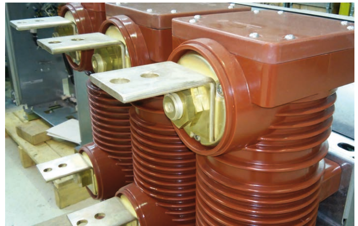
Figure 14. DS1 power connections
